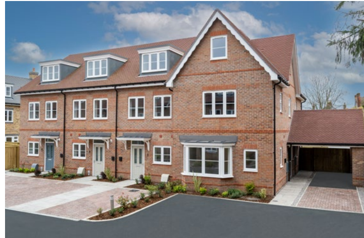
Ashcroft Place, Staines-upon-Thames
